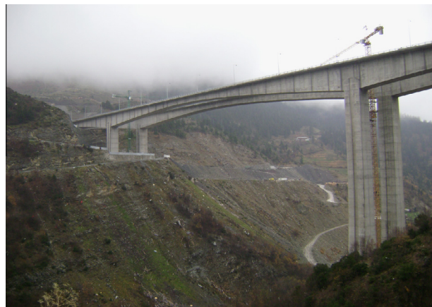
Fig. 1. General view of Metsovo bridge.
