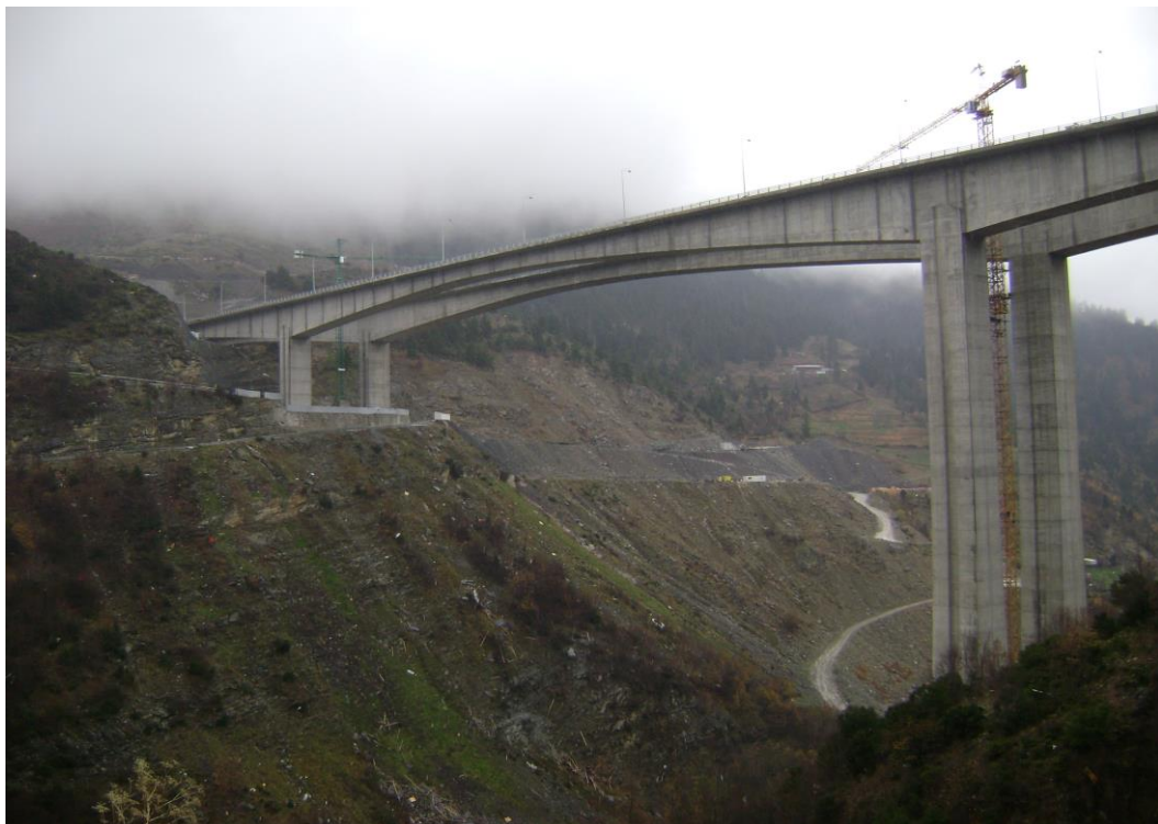
Figure 3.1: General View of Metsovo bridge.
